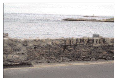
Right: Restored wall at Coliemore
